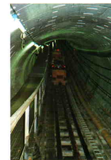
This photograph shows a 5.24 mφ tunnel with an inclination of 15° which was constructed with a downhill grade shield.
